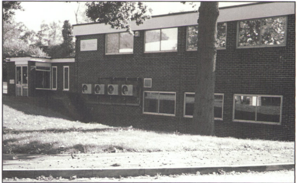
The property at Maxwell Way, Crawley acquired by ROCC
