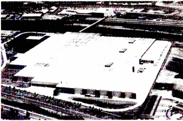
A staggering 1.2 million sq ft, equivalent to 34 Wembley Stadium football pitches forms part of Freemans' warehouse and distribution centre at Peterborough.
