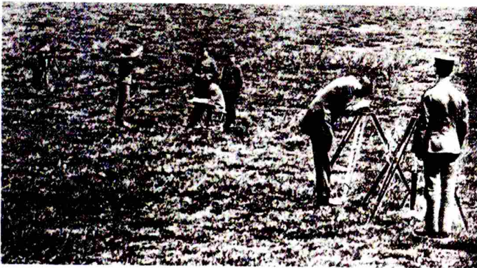
Measuring the length of the Lossiemouth Base, carried out between 1909-1911 by Ordnance Survey surveyors. This base line covering many kilometers was used to test the completion of the triangulation of Britain.
